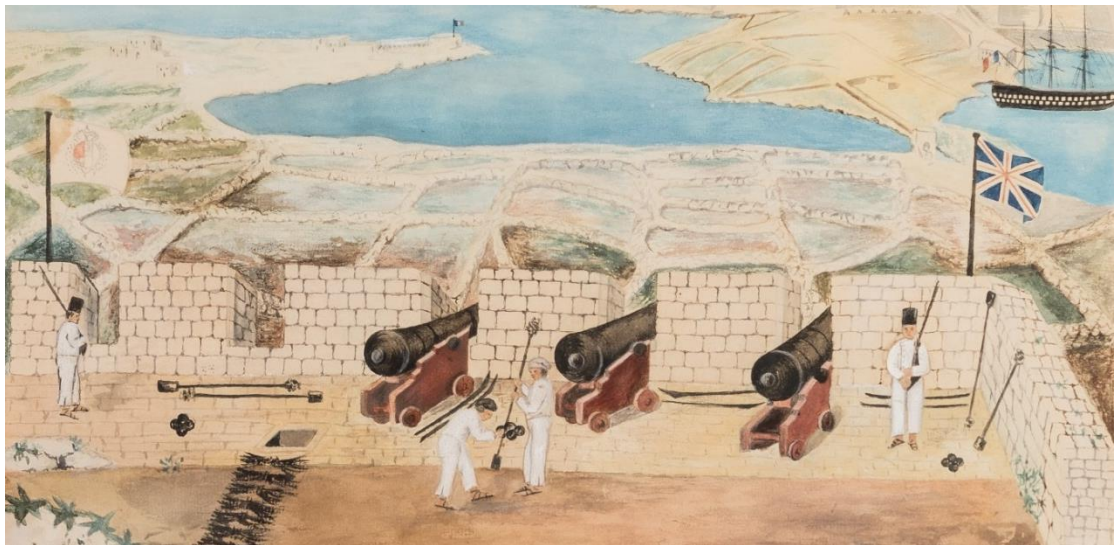
Figure 14 – Maybe the first interpretation of the "Għargħar" Gun Battery, unknown artist (Heritage Malta)
